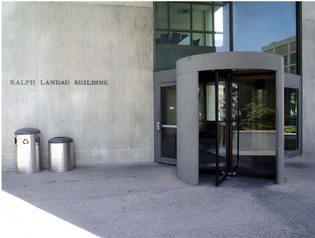
Figure A14. Building 66, corner - Ames Street side.
