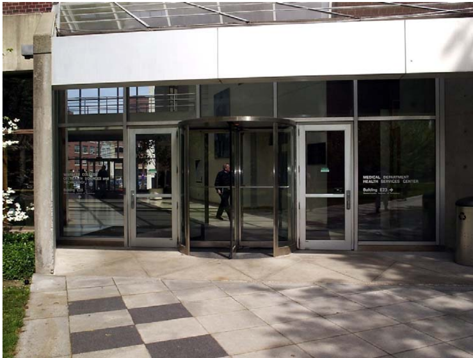
Figure 11. E25(2) doors. This is an example of the standard configuration for a revolving doors set.
