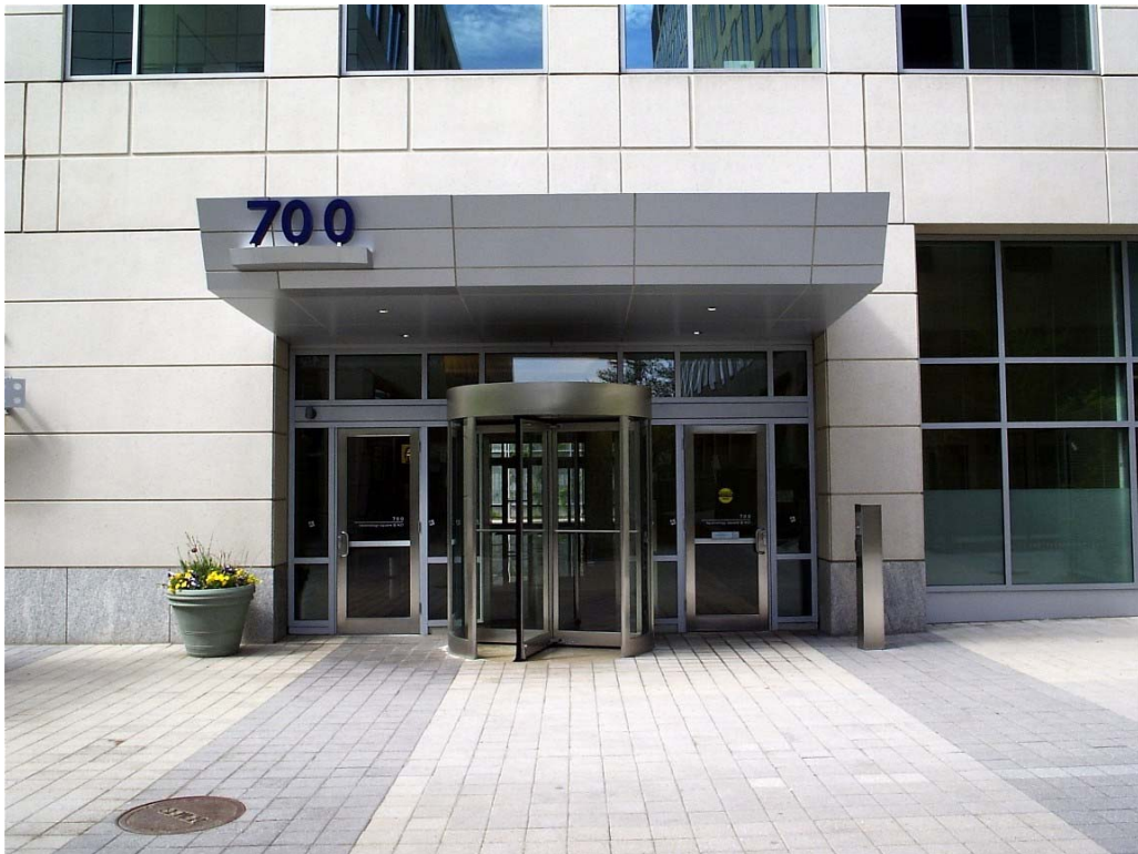
Figure A7. NE48 (700 Tech Square) - Courtyard side.
