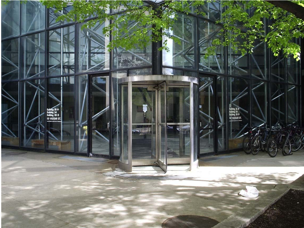
Figure A10. Building 34 -Vassar St. side.
