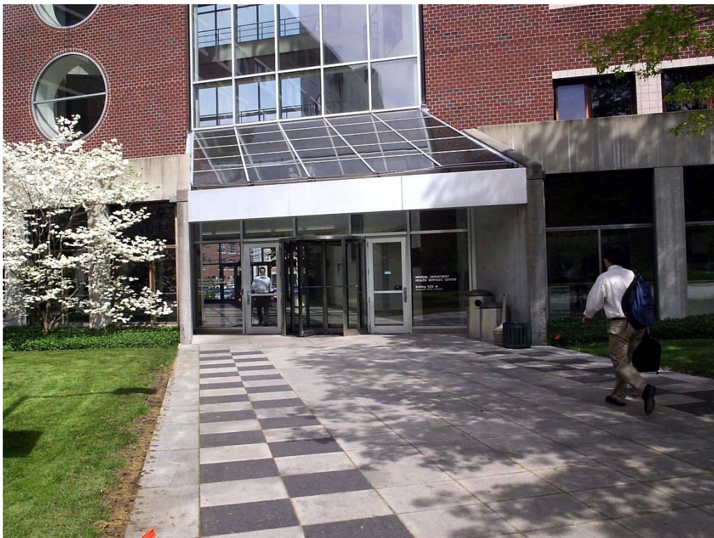
Figure A5. E25 (2) - View from a user approaching from the main campus.
