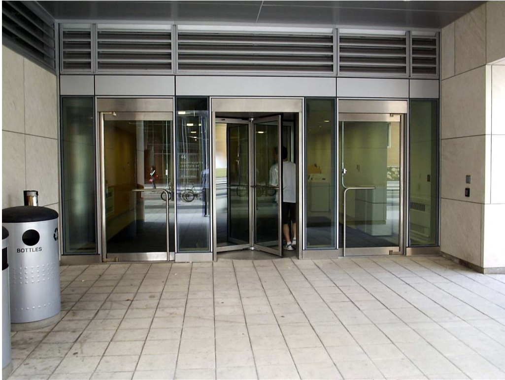
Figure A12. Building 46 (Brain and Cognitive Science Building) - Vassar Street side.
