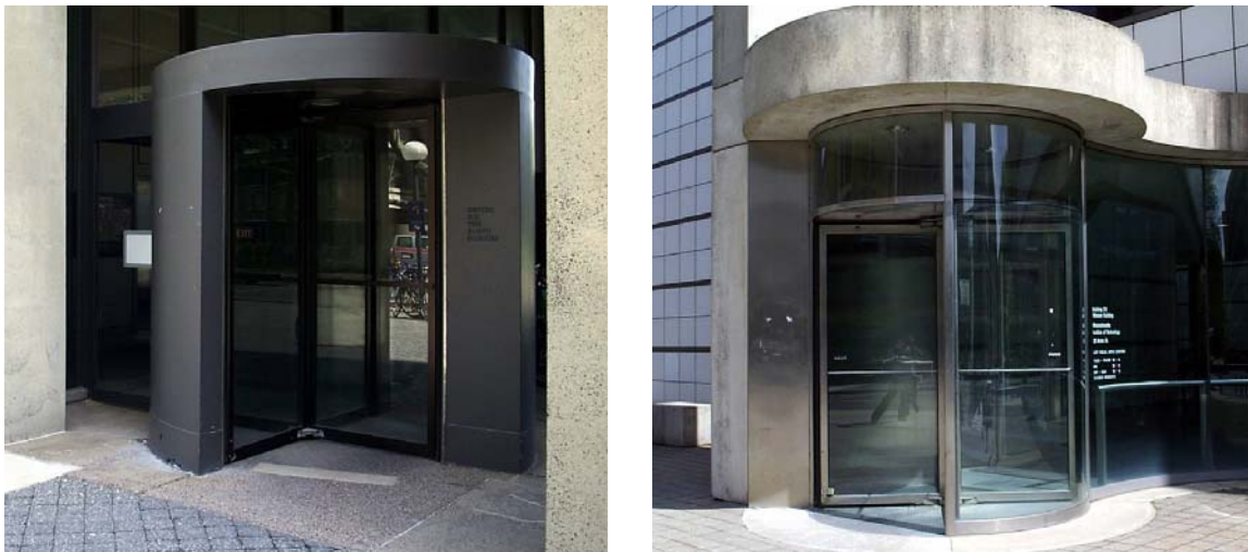
Figure 9. Revolving doors with hidden swing doors. Building 54 (left) and E15(2) (right) have revolving door use rates of over 75%. Swing doors are hidden from approaching users.
